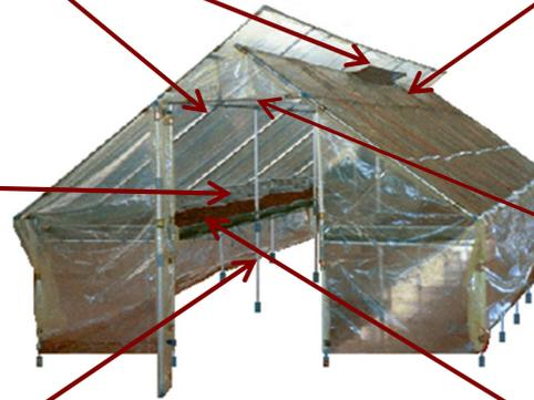
The roof is made of plastic material very resistant to rain, to temperature and to direct and prolonged exposure to the ultraviolet fraction of the solar rays.
